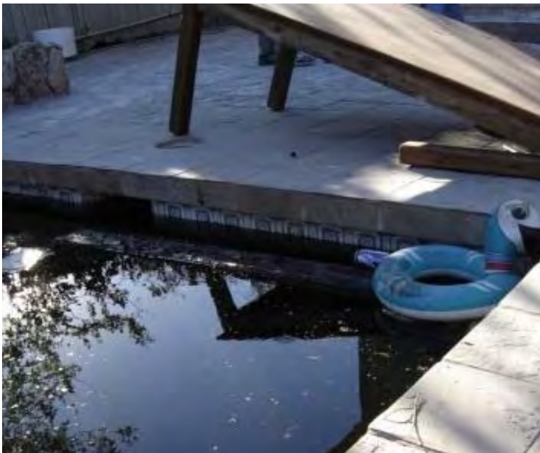
Standing water after Hurricanes Katrina and Rita
